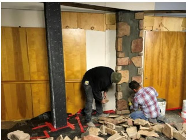
Left: Crews from Peak Stucco and Stone begin attaching stonework to the new set in Candelaria 1315. The wood pillars were covered with mesh and heavy paper before grout and stone were applied. Peak donated approximately \$5,000 worth of stone and labor for the sets.
