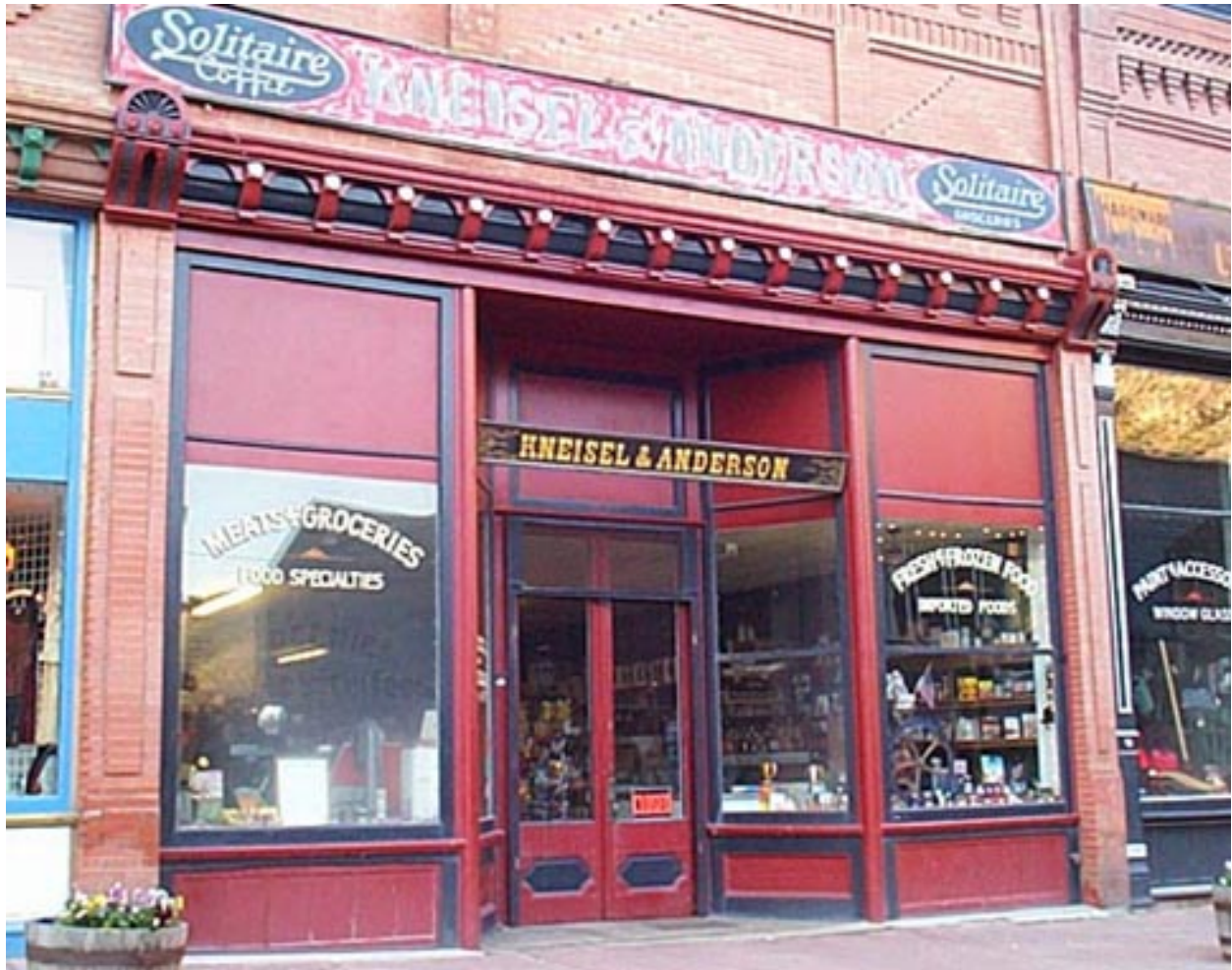
Kneisel and Anderson Grocery and Hardware store
