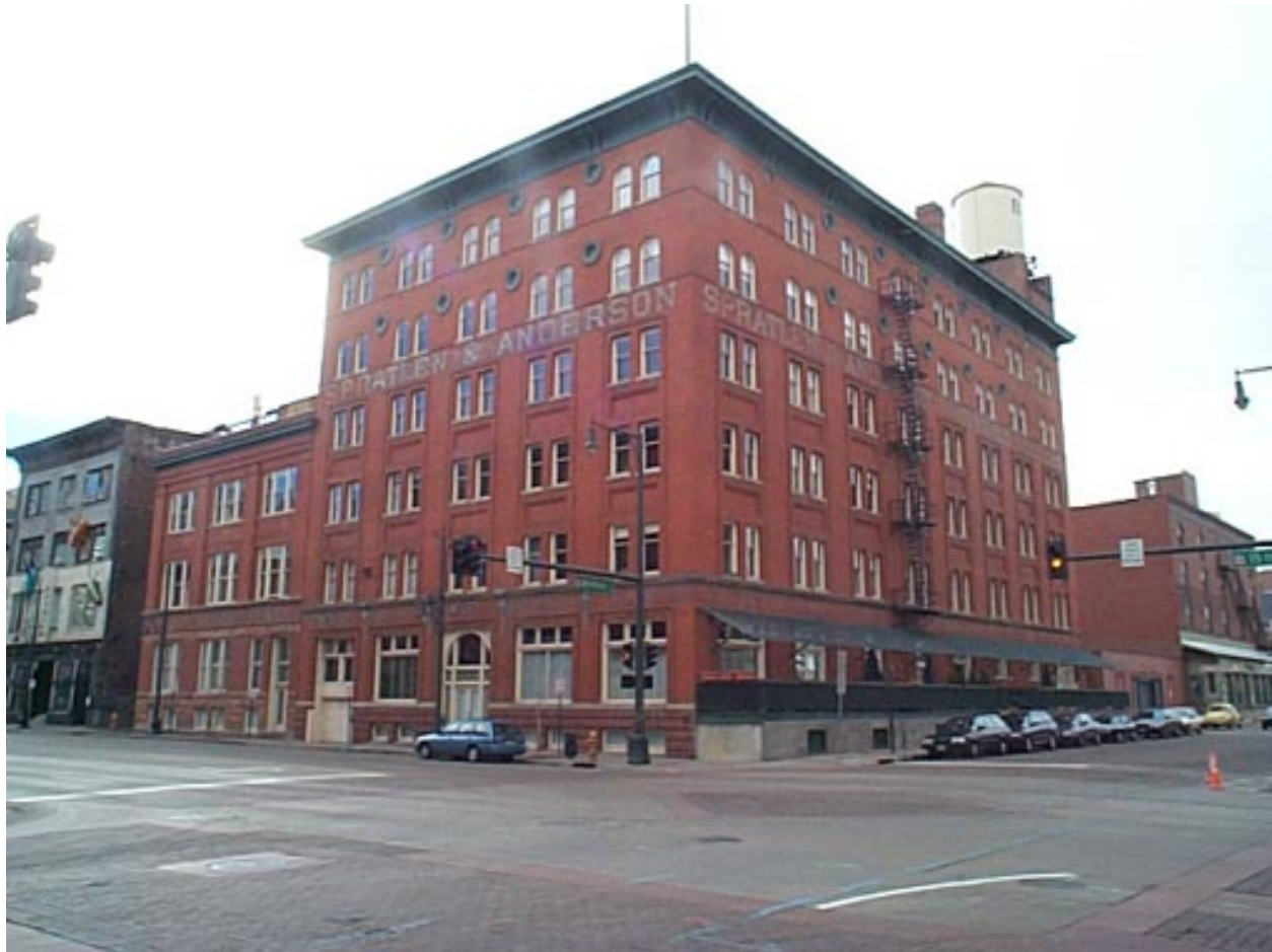
The Spratlin-Anderson Warehouse
