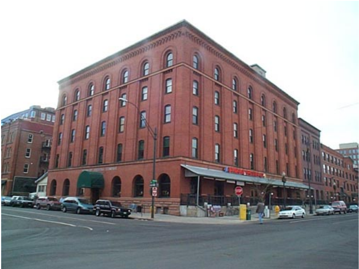
J.S. Brown Mercantile building
