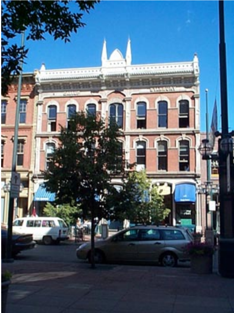
The Gallup-Stanbury building
