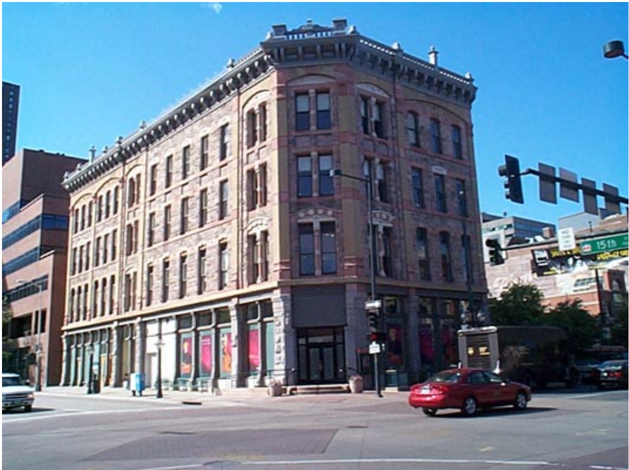
The Clayton building
