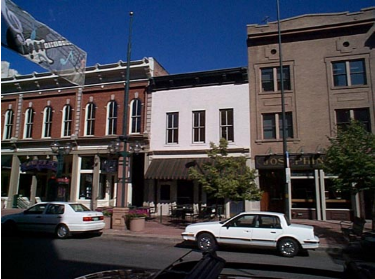
The Looms building
