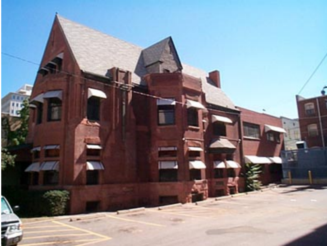
Colorado State Archives building
