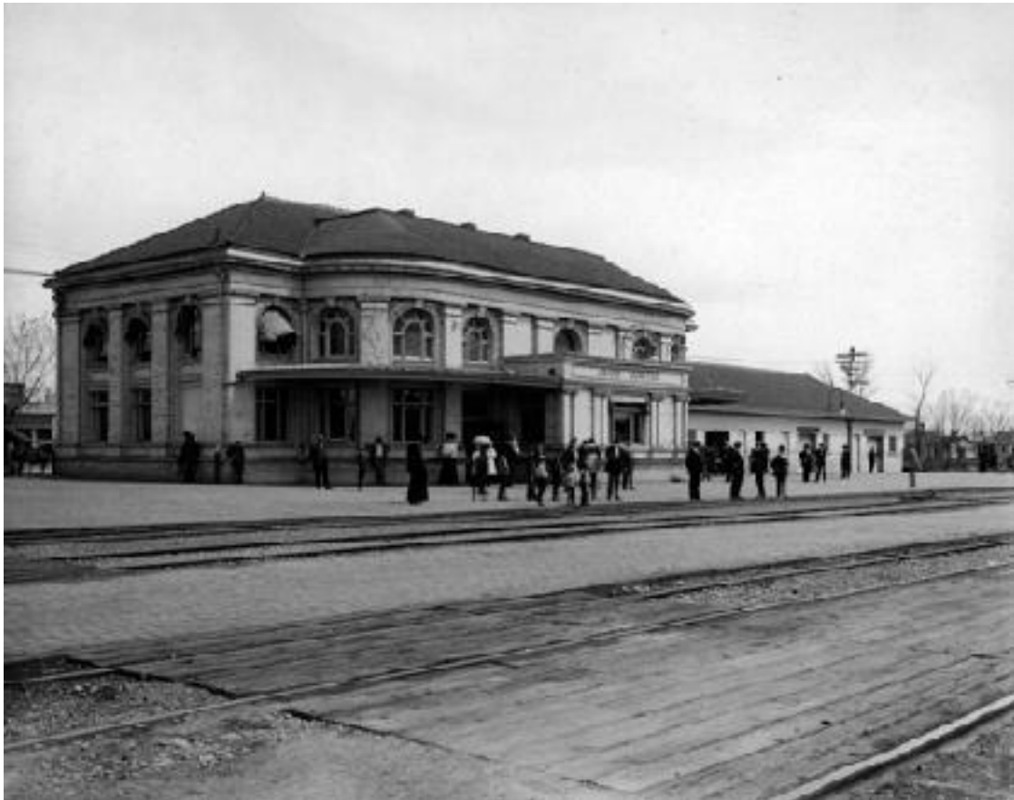
Grand Junction modern Railroad Depot
