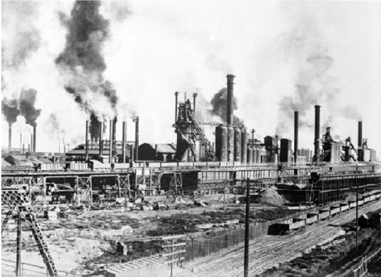
Steel Mill in Pueblo, Colorado
