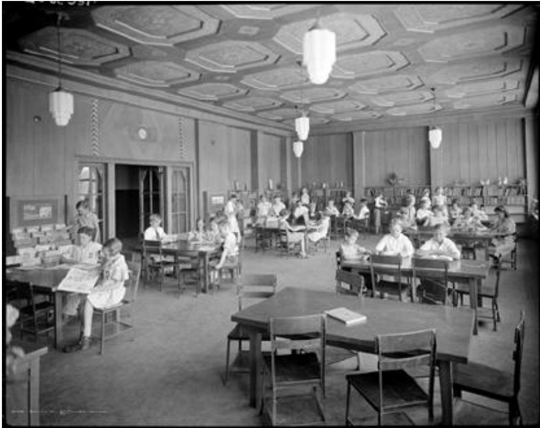
School library at Steele Public School
