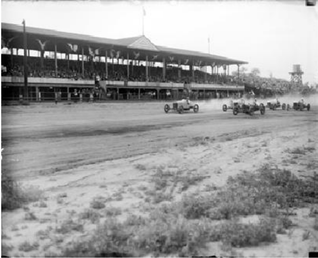
Overland Park in Denver
