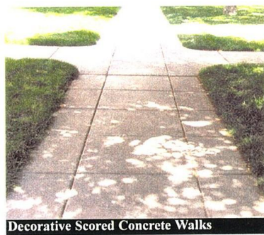
Decorative Scored Concrete Walks
