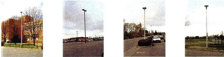
PARKING LOT LIGHTING
