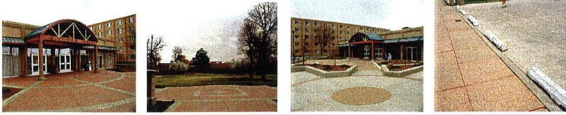
CRANFORD PAVEMENT - COLORED CONCRETE
