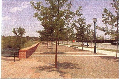
Low Water Use Streetscape
