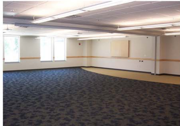
Recycled content carpet and FSC certified wood products installed.
