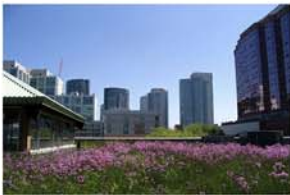
IDc1.2: Provided open space area greater than twice the are of the building footprint.
